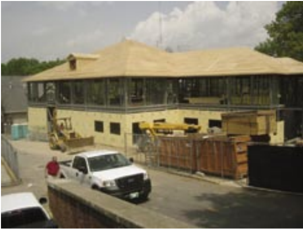
House renovations as of early April 2007.
